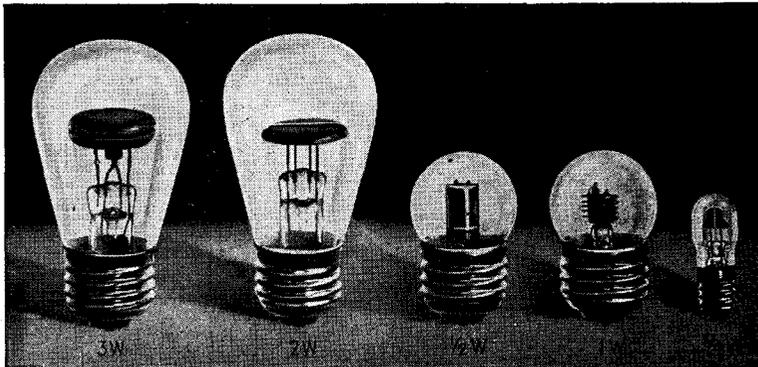
FIG. 2-21. Photographs of several low-capacity glow lamps. (General Electric Co.)
